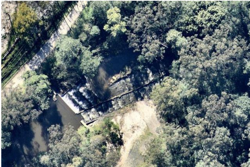
Figure 3.3 Ourimbah Creek Weir and fishway (obtained from NearMap: captured on 18 August 2022)
