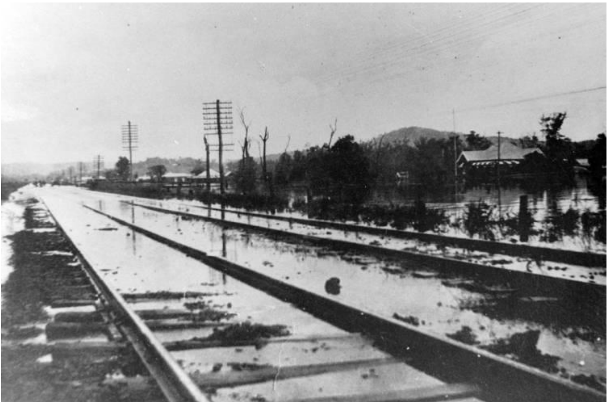
Figure 1.3 Northern railway line just north of Tuggerah Station covered by flood waters, Wyong 1927. Courtesy of Central Coast Council
